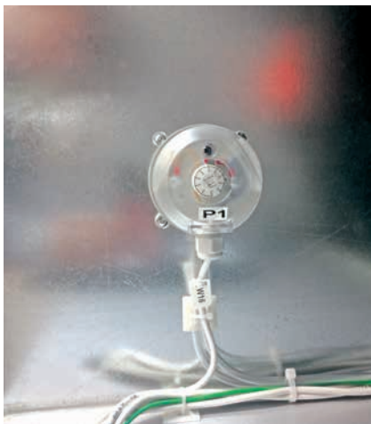
Figure 49: Differential pressure switch for fresh air or extract air filters.
