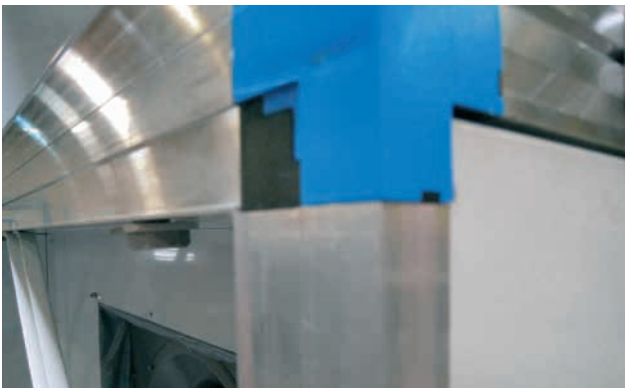
Figure 14: Apply self-adhesive EPDM rubber sealing tape with a 20 x 8 mm cross-section (supplied with the air handling unit) onto the contact front faces (housing frame), when connecting the sections with aluminium profile.
