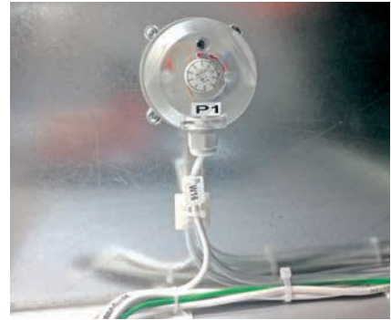
Figure 50: Differential pressure switch for fresh air or extract air filters.
